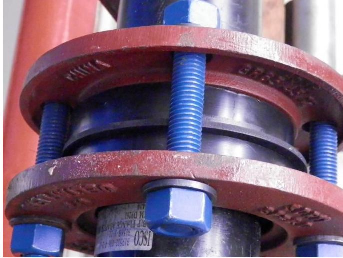
Figure 1 (3" 150lb HDPE with metal flange backer)
