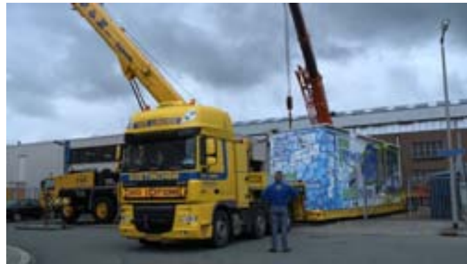
The Nedstack 1 MW fuel cell PEM Power Plant being loaded onto the low loader truck, ready to deliver to the Solvay chlorine plant in Lillo, near Antwerp in Belgium.
