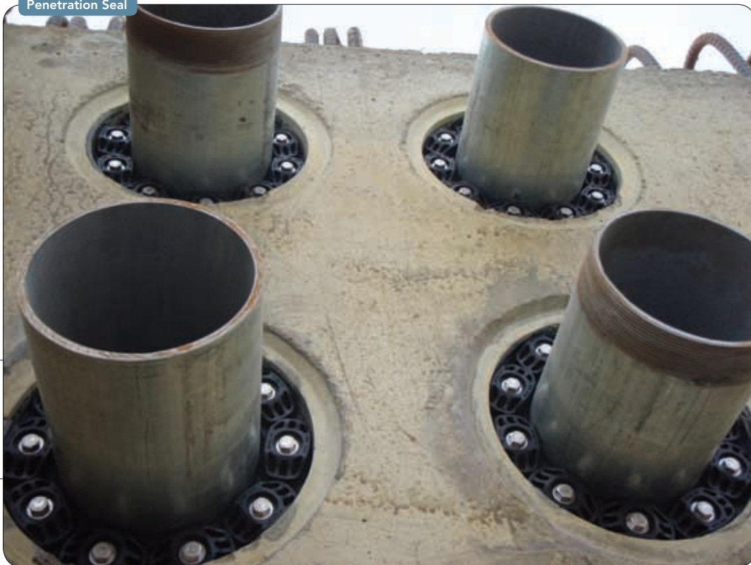
Figure 2. Modular line of seals are used when pipes go through walls. Source: Garlock Sealing Technologies.
