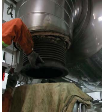
The installation of reinforced ceramic sheet gasketing in the exhaust system of the 225-ft. (68.6m) yacht Attessa after spiral-wound graphite gaskets oxidized and caused leaks.
