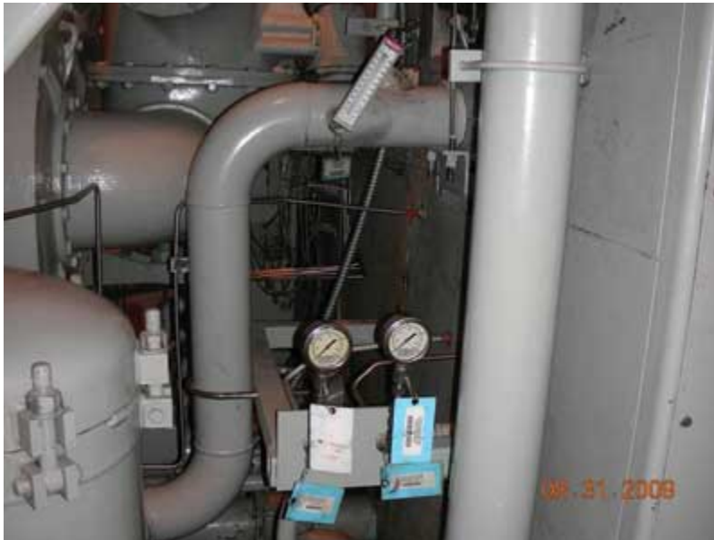
Pre-expansion joint installation
